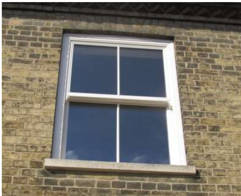
An example of high quality UPVC windows has been used in the unlisted manse on Gracious Street.
