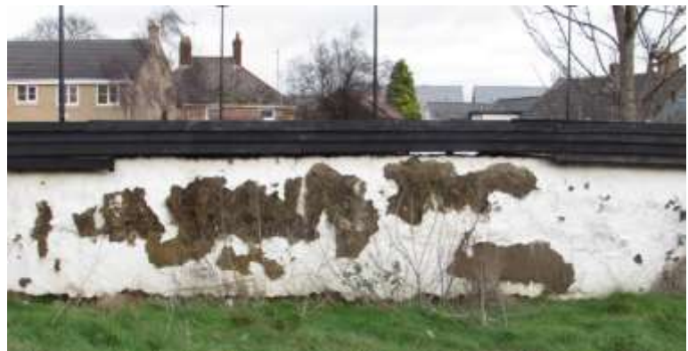
Scaffolding and deteriorating mud walls
