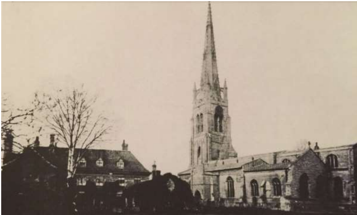
Manor House sits adjacent to St Mary's Church and historically the two were viewed together from Station Road (photo; Whittlesey Museum).
