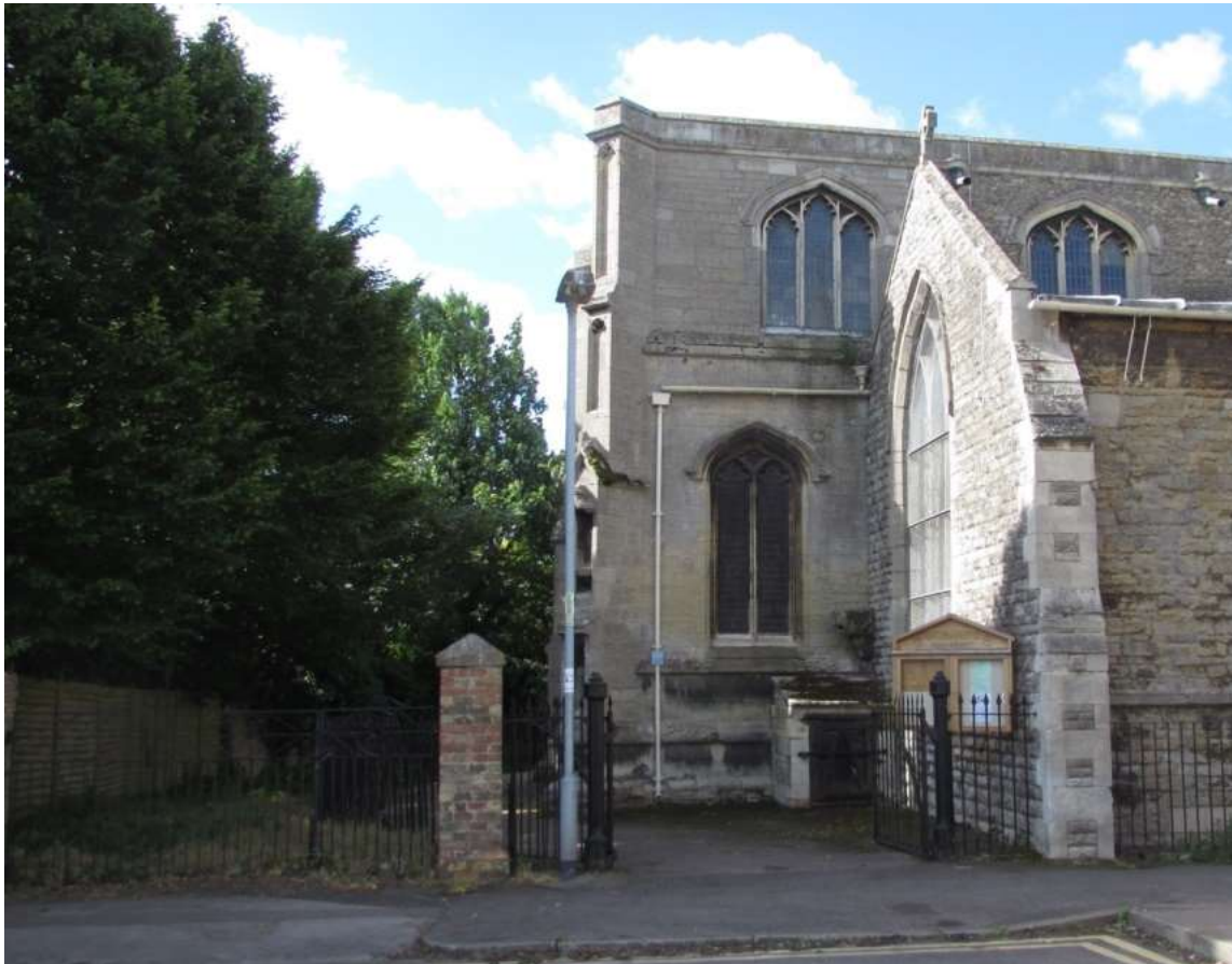
The utilitarian lighting column to the entrance to St Mary's Church is an example of poor public realm detail and detracts from the setting of the church.
